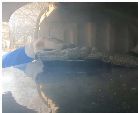
Application of PED-Pad fire suppression pillow ...
